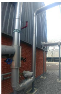
TANK INFILL LAGGING
