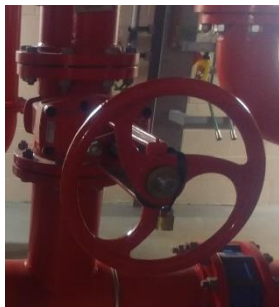
DIESEL FLOW VALVE
