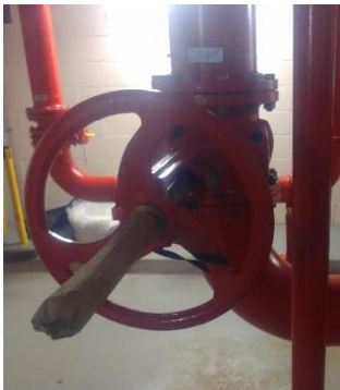
DIESEL DELIVERY VALVE
