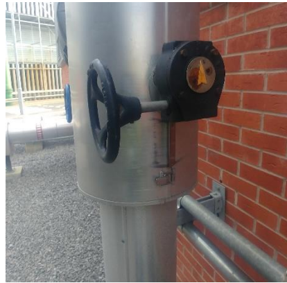
TANK INFILL VALVE
