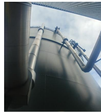
TANK INFILL LAGGING
