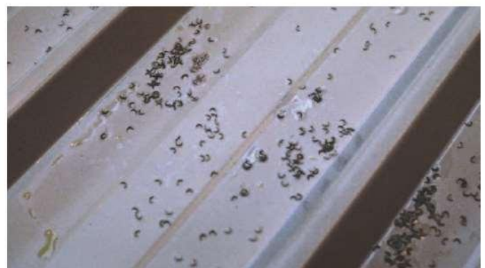
Swarf left on a roof.
