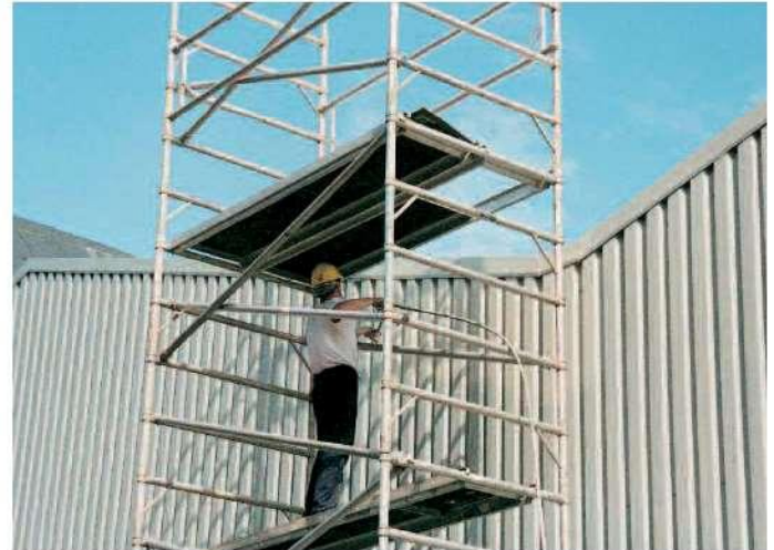
Wall cladding being over-painted.
